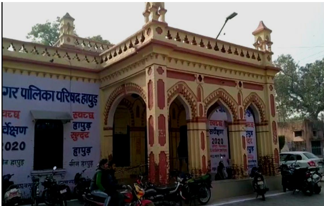
Figure 16. Nagar Pallika building, erstwhile Haveli of Chaudhary Prannath and his daughter Mangla
