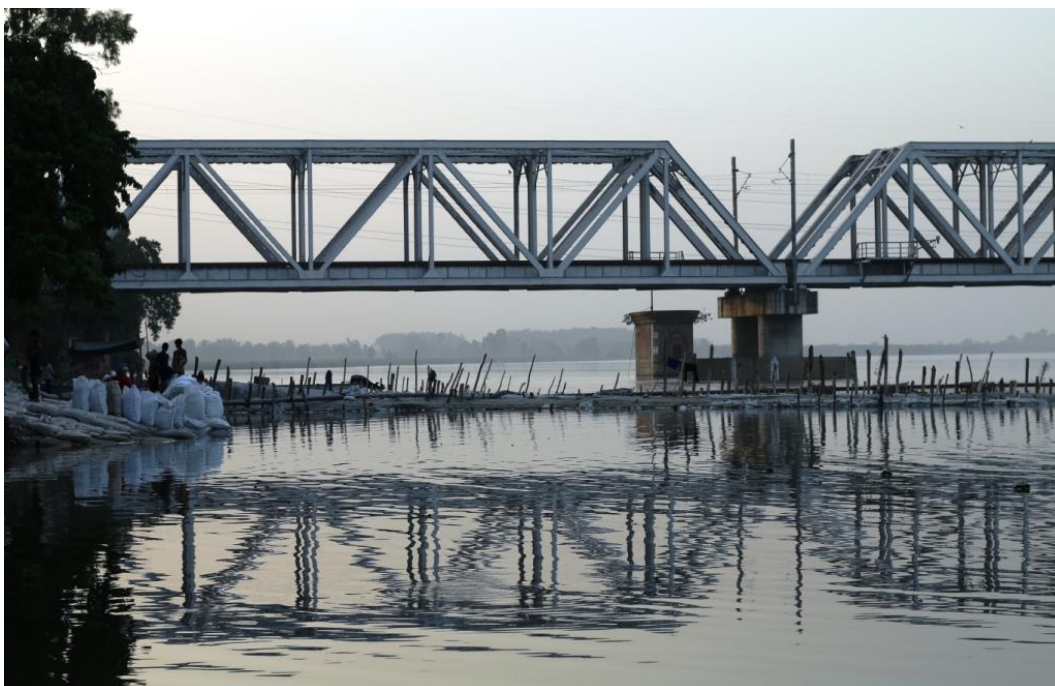
Figure 11. View of the old iron bridge
